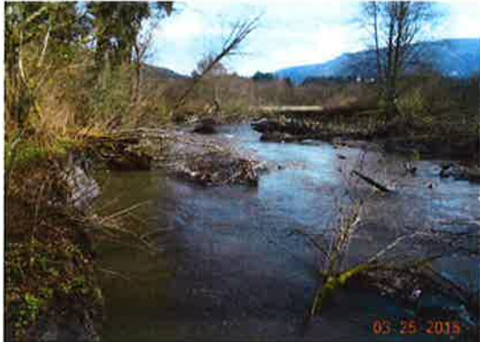
Photo 1 - View north showing active channel and cut left bank. Note erosion and recruitment of woody debris into channel.
